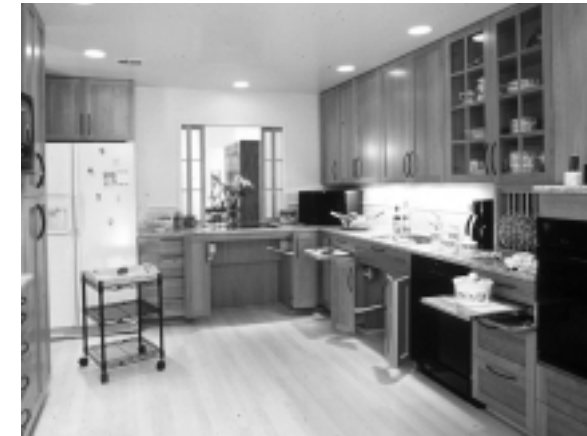
This kitchen provides ample work space, a raised dishwasher and lowered cooking surfaces.*
